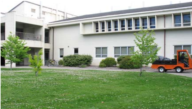
Character of the new Math and Science building should reflect the existing architectural styles.
