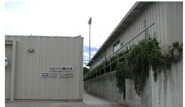
The existing pool changing rooms are planned to be removed and replaced with a new building on the east side of the pool.
