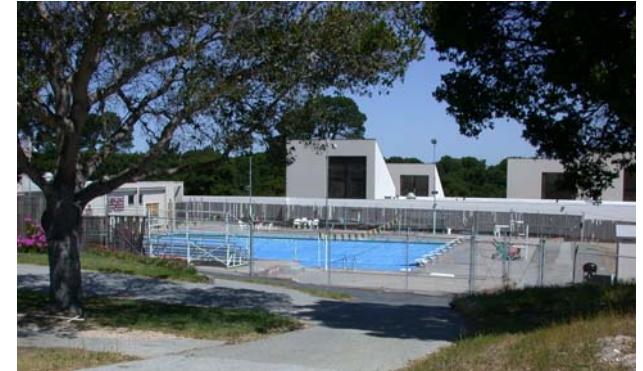
The swimming pool is being replaced.
