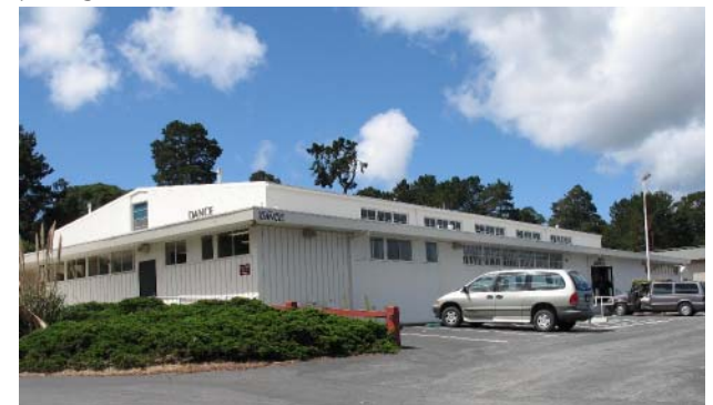
The Old Armory should be renovated to house the Nursing program.
