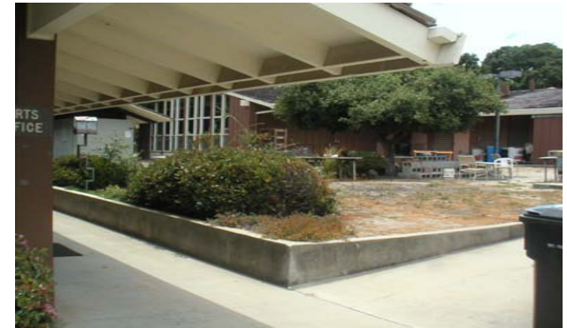
Creative Art courtyards are appropriately scaled to the surrounding buildings.
