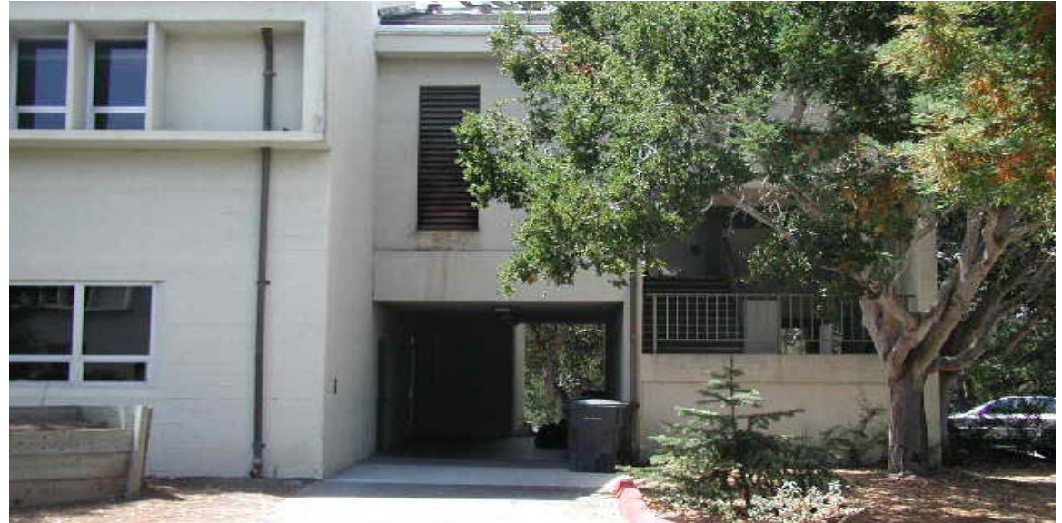
Entries should be clearly visible from pedestrian paths and not hidden behind blank walls or structures.
