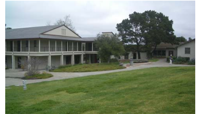
The existing buildings have exterior verandas typical of the Monterey Style.
