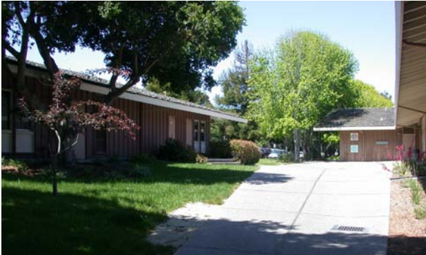
The Creative Arts buildings are primarily post and beam construction.
