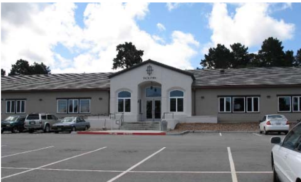
The Plant Services building is one of the most recently constructed buildings on campus.
