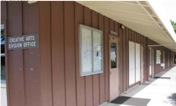
Exterior corridors extend the length of the Creative Arts buildings.
