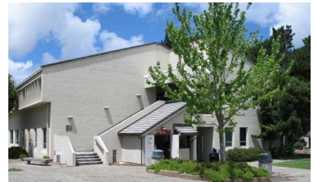
The Social Sciences building bridges between the Business and Humanities Cluster and the Math and Science Quad.
