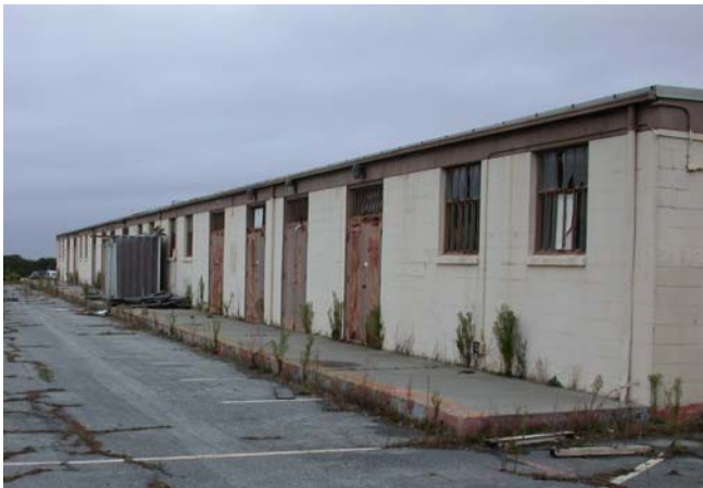
Existing parking lot and west facade of Building #4464
