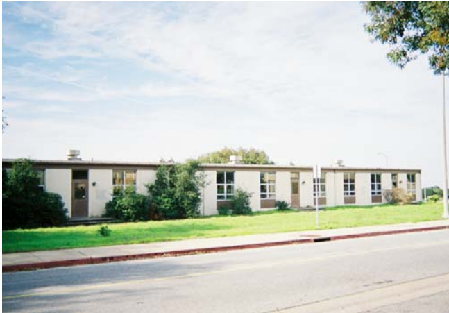
East facade of Building #4464
