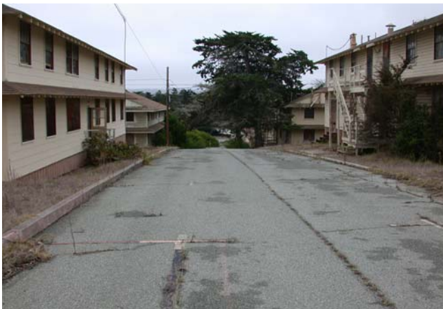
Existing barracks (future parking site) west of 11th Street
