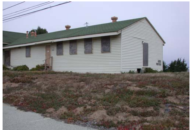
South facade of Building #T-2898
