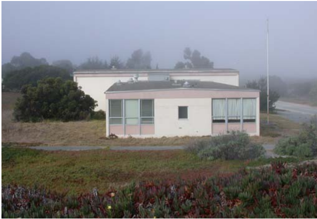
Looking west at Building #4465 from the upper parking lot
