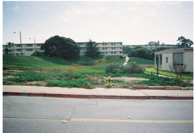
Looking south from Col. Durham Road, Building #4465 at right
