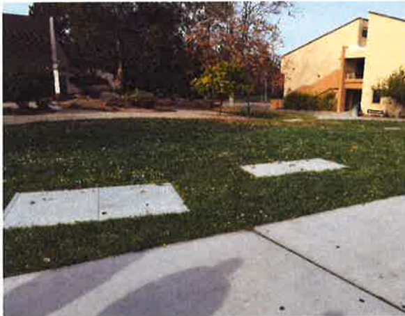
Figure 81: Un-mowed turf and goose droppings on underground services cover outside Physical Science Building.
