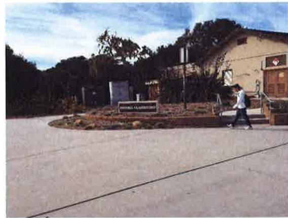
Figure 55: Pavement around General Classrooms Building
