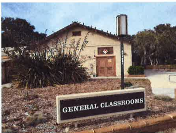
Figure 54: External facade of General Classrooms Building
