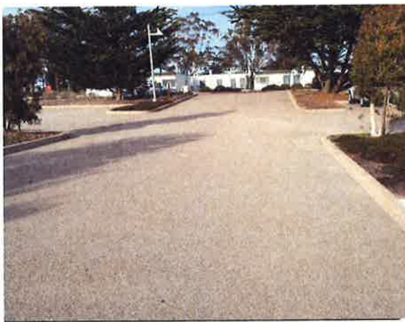
Figure 66: Asphalt at Marina Center
