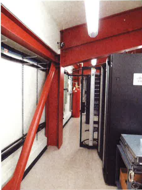
Figure 60: Seismic retrofit detailing in server room
