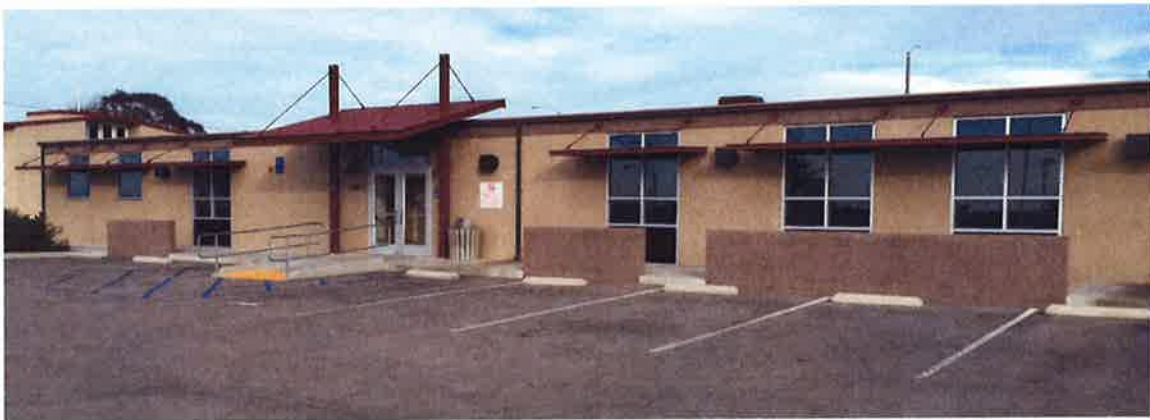
Figure 102: Asphalt and front elevation at Seaside Public Safety Training Center
