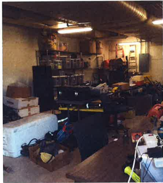
Figure 3: Equipment service and storage room at Seaside Public Safety
