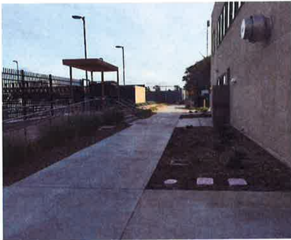
Figure 70: New pavements, reclaimed irrigation control boxes and landscape at front entrance of Gym
