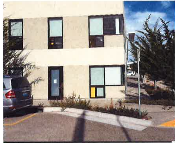
Figure 50: Southeast corner elevation view of Student Services Building without awnings or sunshade elements
