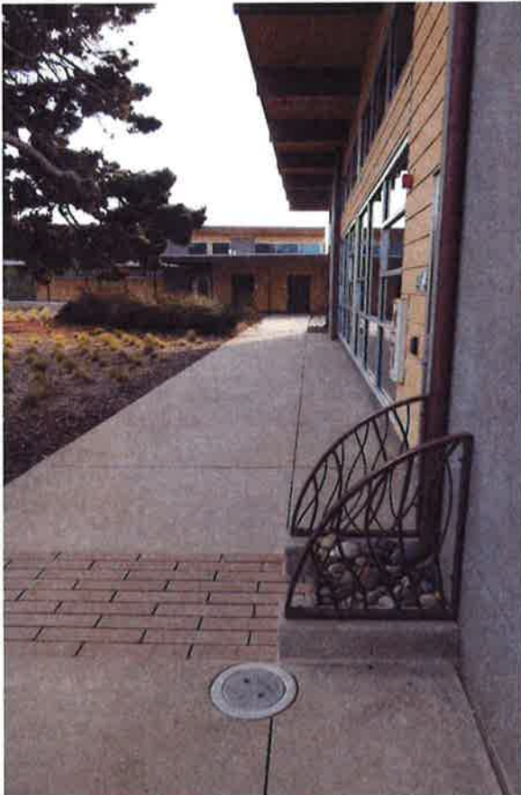
Figure 39: Bioswale detention basin, pavements and landscape at Marina Center
