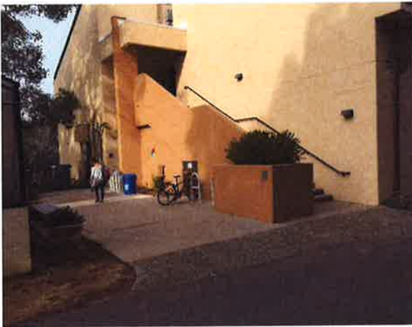
Figure 58: External facade & pavement at Life Sciences Building
