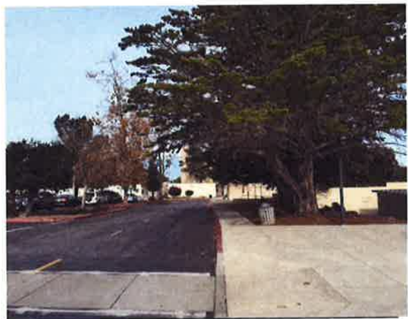
Figure 67: Asphalt in Car Lot C adjacent to Facilities Building
