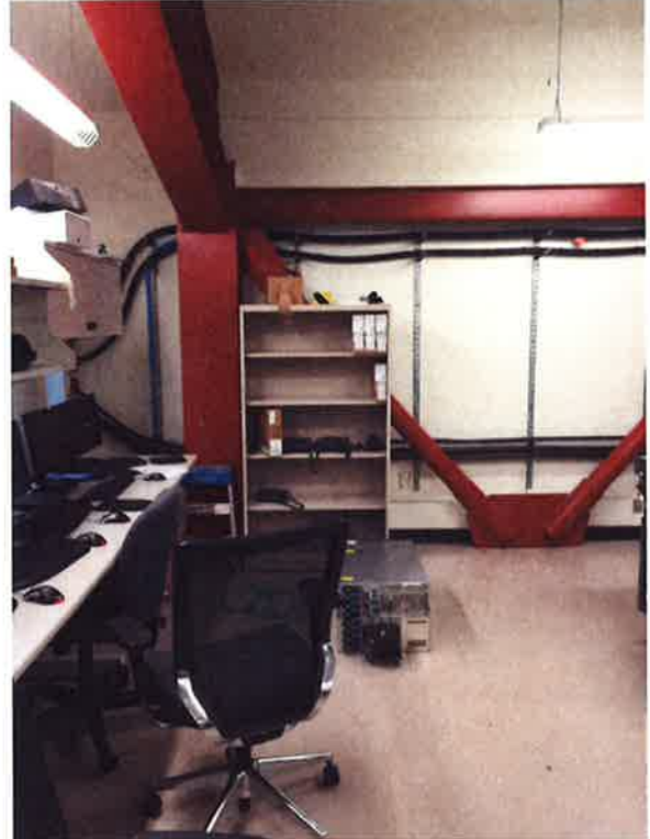
Figure 61: Seismic retrofit detailing in server room
