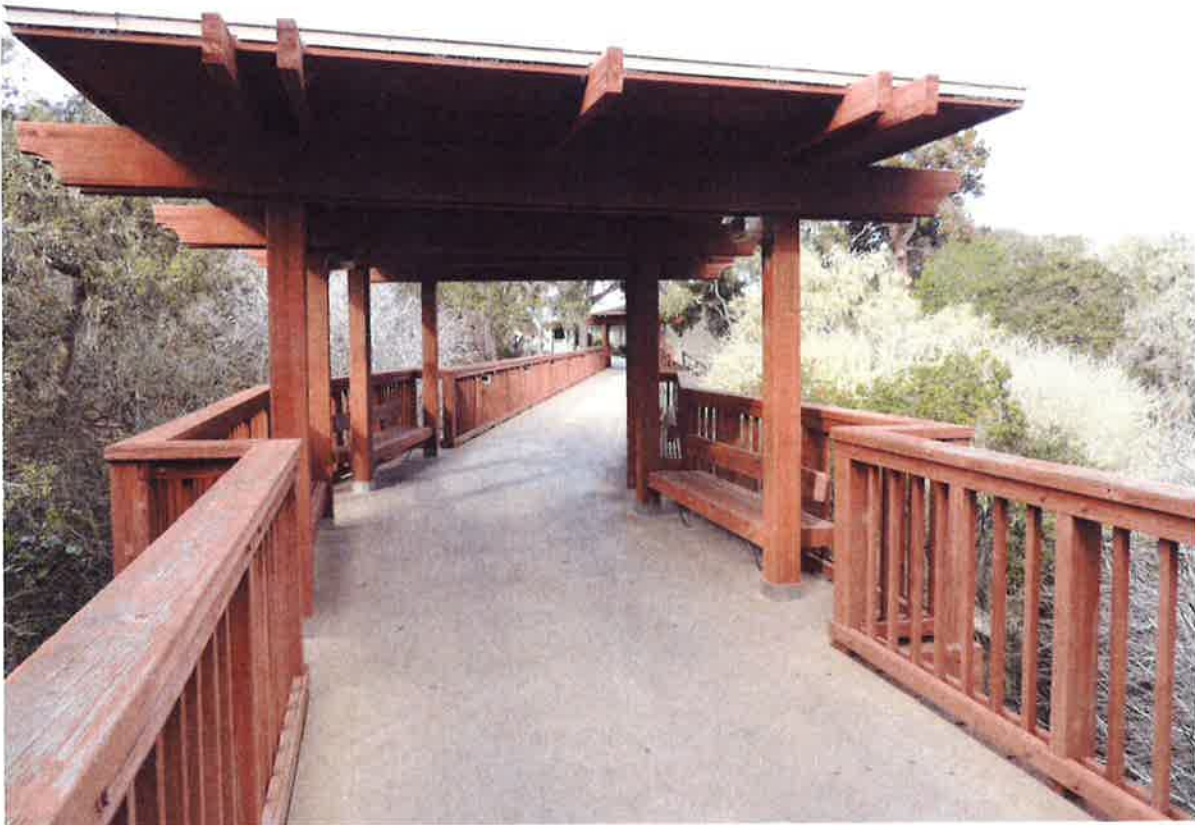
Figure 74: Bridge walkway & halfway viewing point
