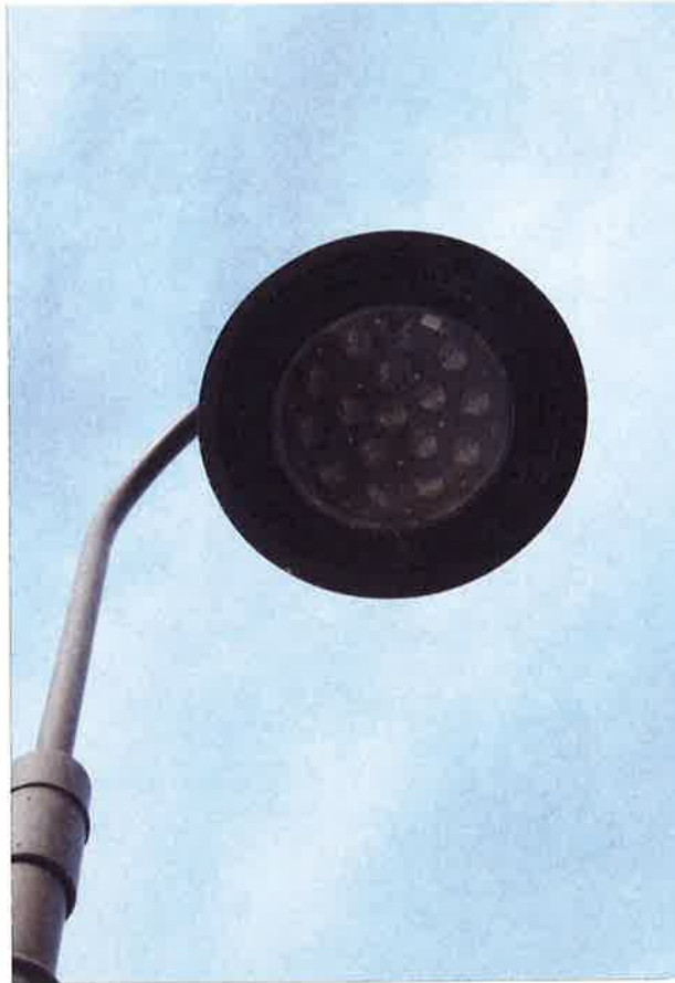
Figure 31: Exterior "Spanish Lamps" retrofitted with LED lighting
