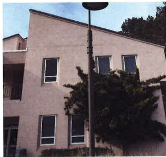
Figure 59: External facade of Social Science Building
