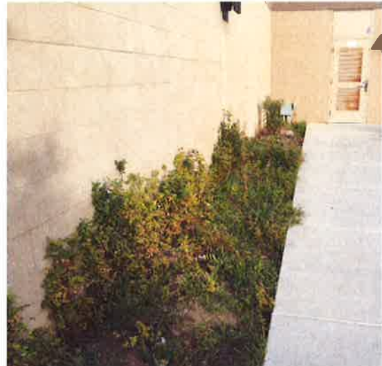
Figure 105: Shrub beds at Seaside Public Safety Training Center
